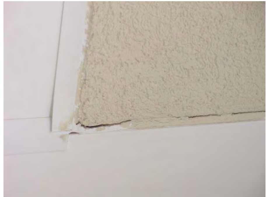
4. Sealant joint cracking at EIFS - composite trim detail
