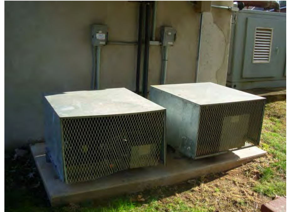
18. Condenser-compressor units serving kitchen refrigeration
