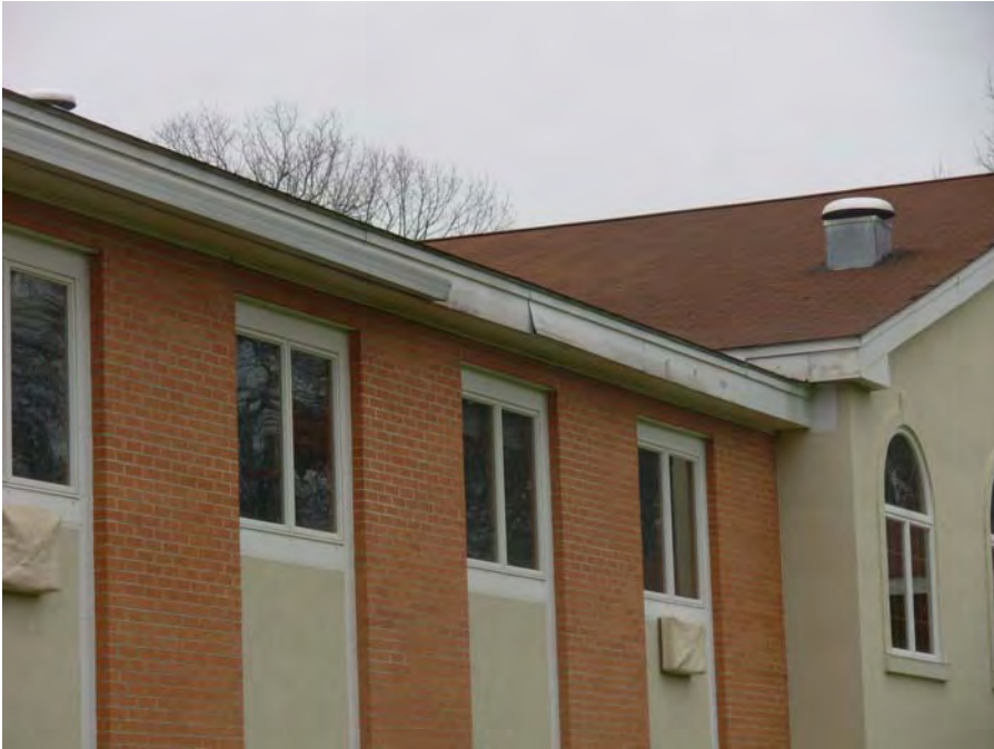
5. Gutter and fascia damage at rear of building
