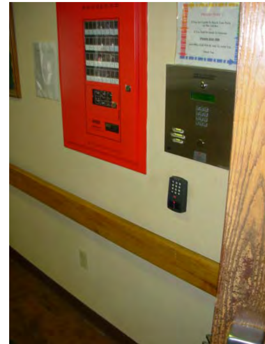
20. Fire detection-monitoring panel and intercom call system
