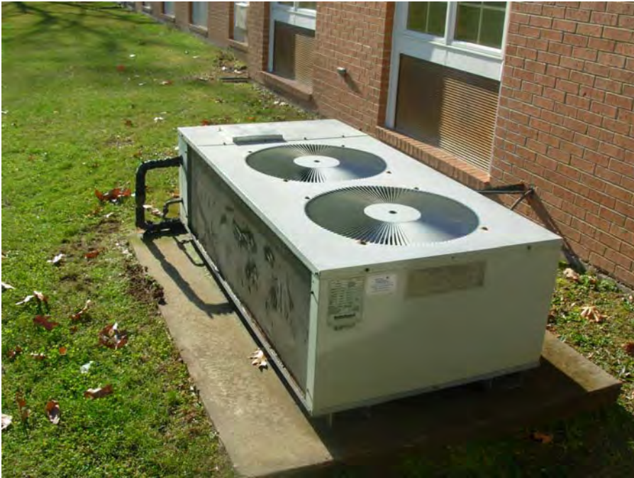
17. Condenser-compressor unit serving central core HVAC
