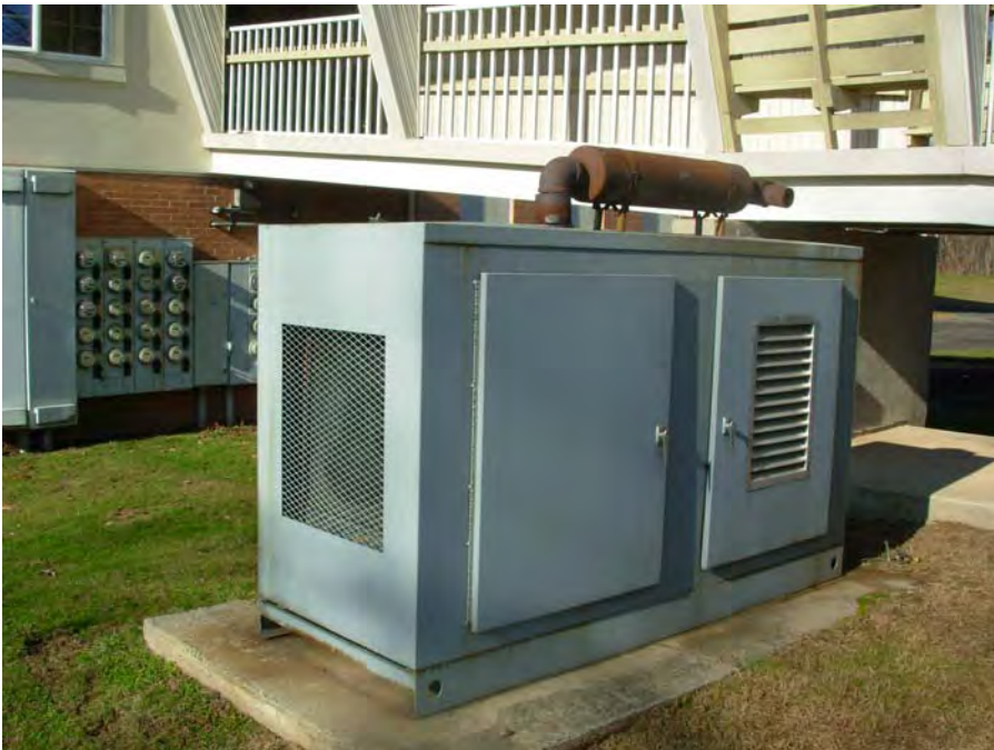
19. View of the emergency generator
