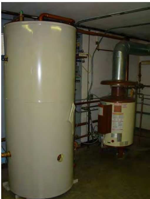
15. DHW boiler and storage tank
