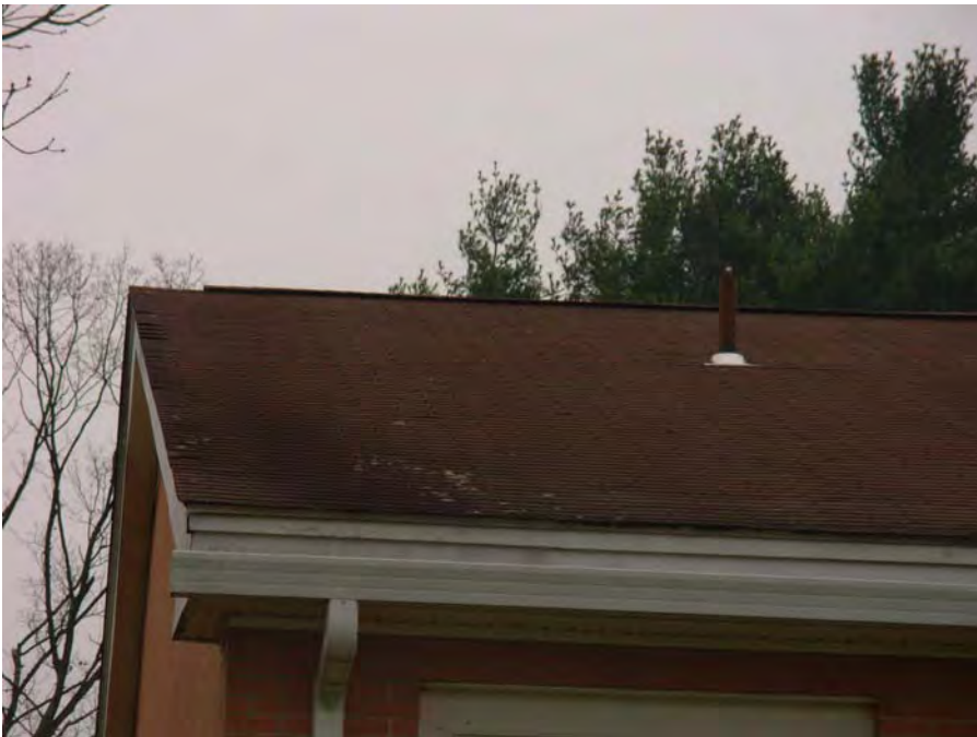
7. View of the main building's roof, note decking deflection
