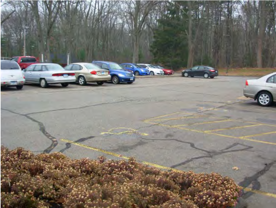
1. Pavement cracking and settlement at main parking area
