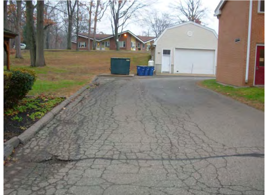
2. Paving settlement and cracking at trash hauler drive lane
